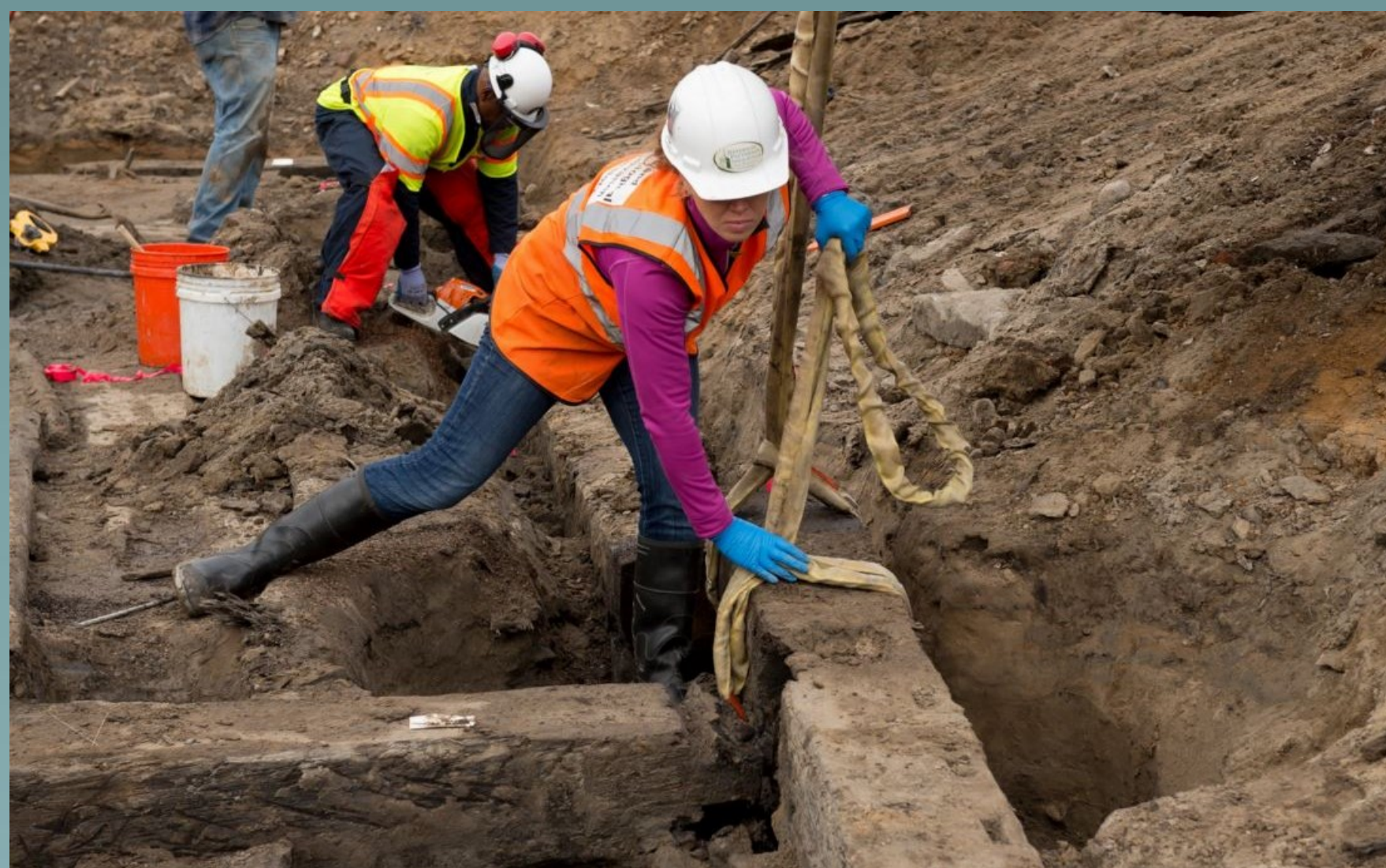
Figure 2. MAC Lab Conservation staff rigging timbers for crane lifts.
